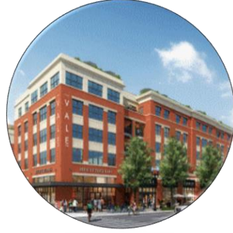
The Vale at Walter Reed Office: Washington Status: In Development City: Washington, DC 301 units
